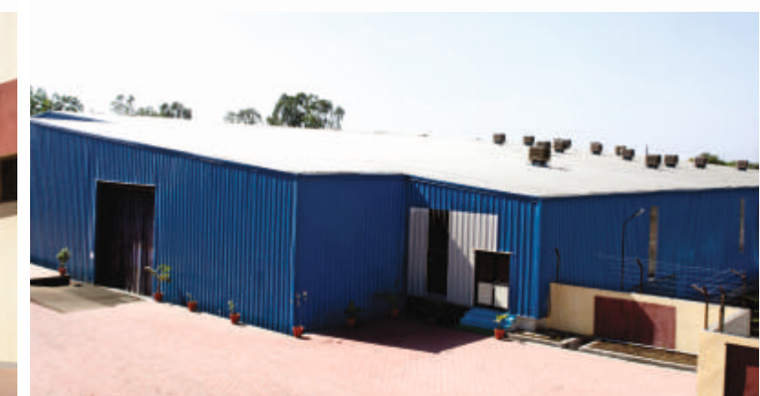
BOOSTER & OPENWELL / MONOBLOCK PLANT
